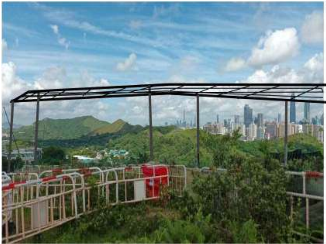
The installation of a shaded net
