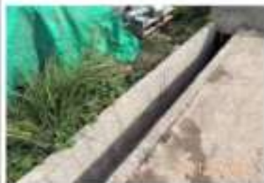
By main contractor at KNP site
