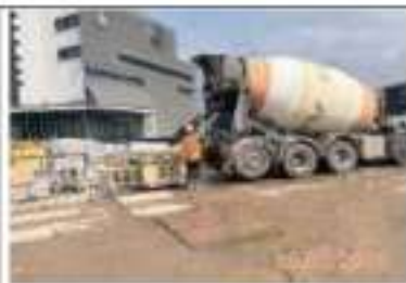
By subcontractor at KNP site
