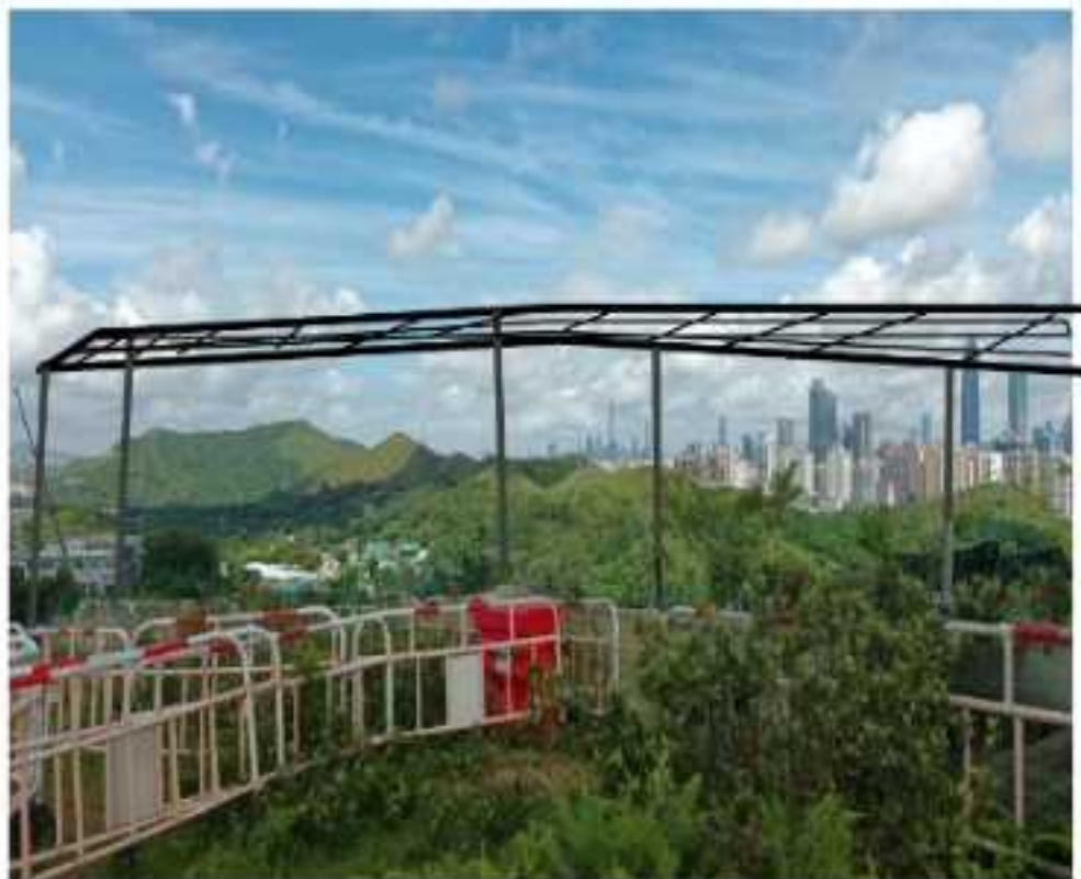
The installation of a shaded net
