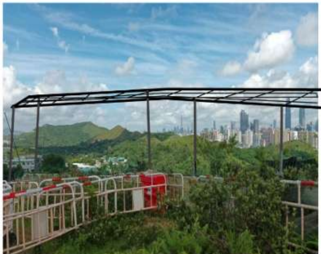
The installation of a shaded net
