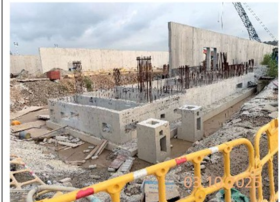
By subcontractor at KNP site
