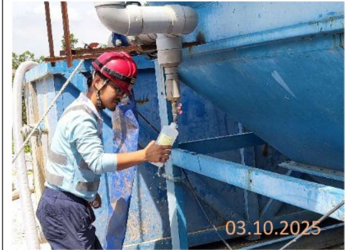
By main contractor at KNP site
