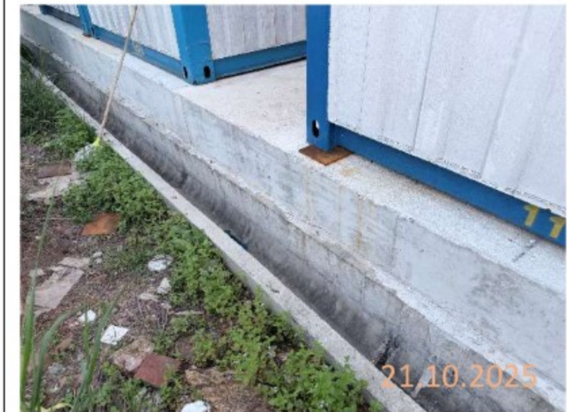
By main contractor at KNP site
