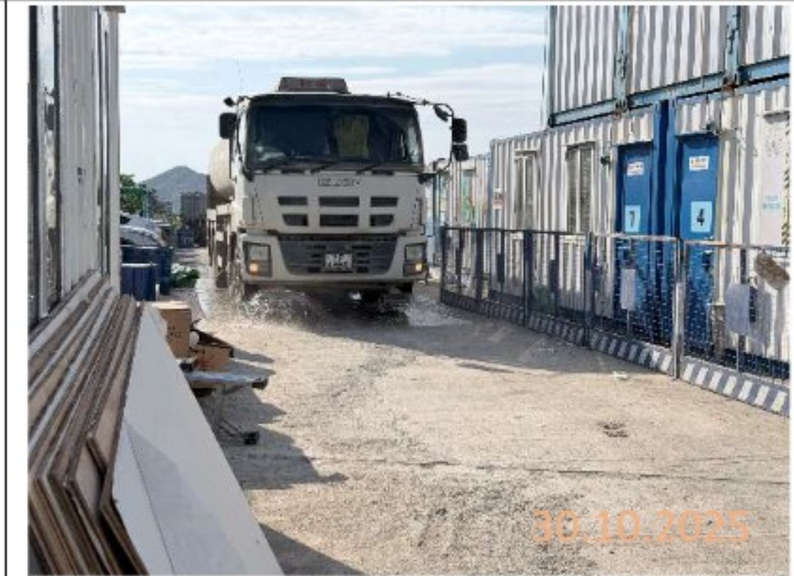
By subcontractor at KNP site
