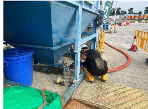
By main contractor at KNP site
