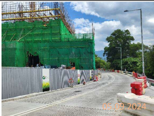
By main contractor at KNP site
