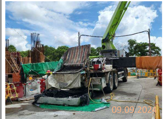
By subcontractor at KNP site
