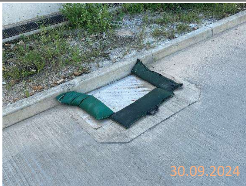
By main contractor at KNP site
