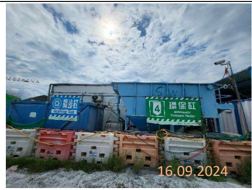
By main contractor at KNP site
