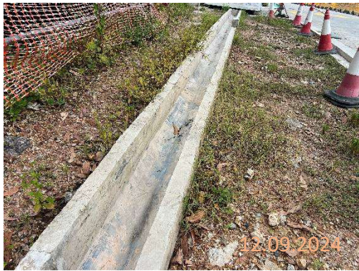
By main contractor at KNP site
