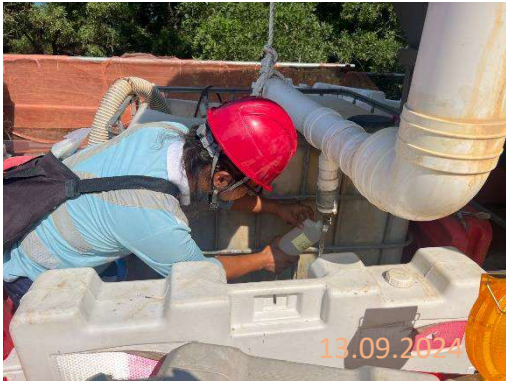
By main contractor at KNP site
