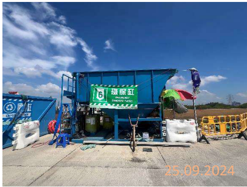
By main contractor at KNP site
