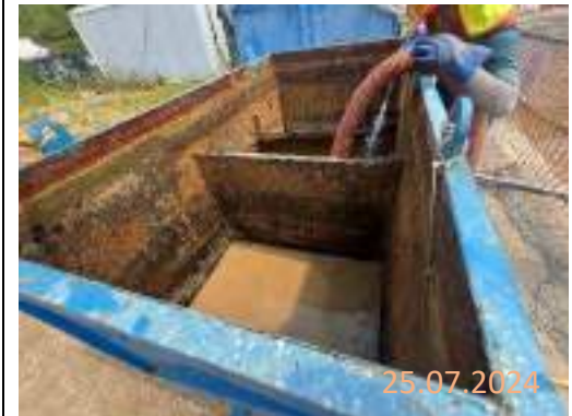
By main contractor at KNP site
