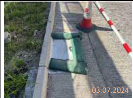
By main contractor at KNP site
