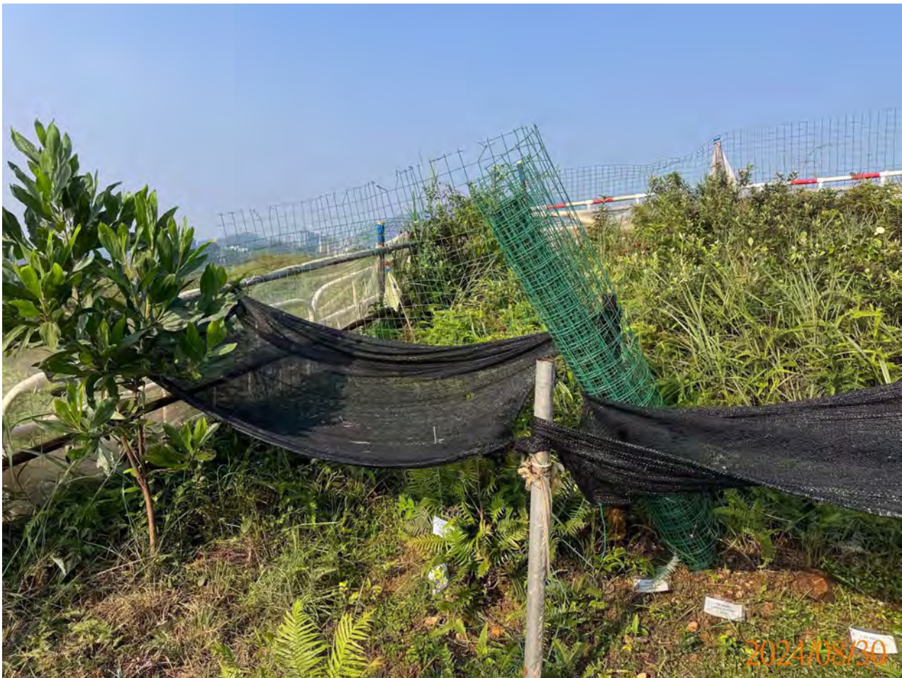
Replacement of protection fence (1)
