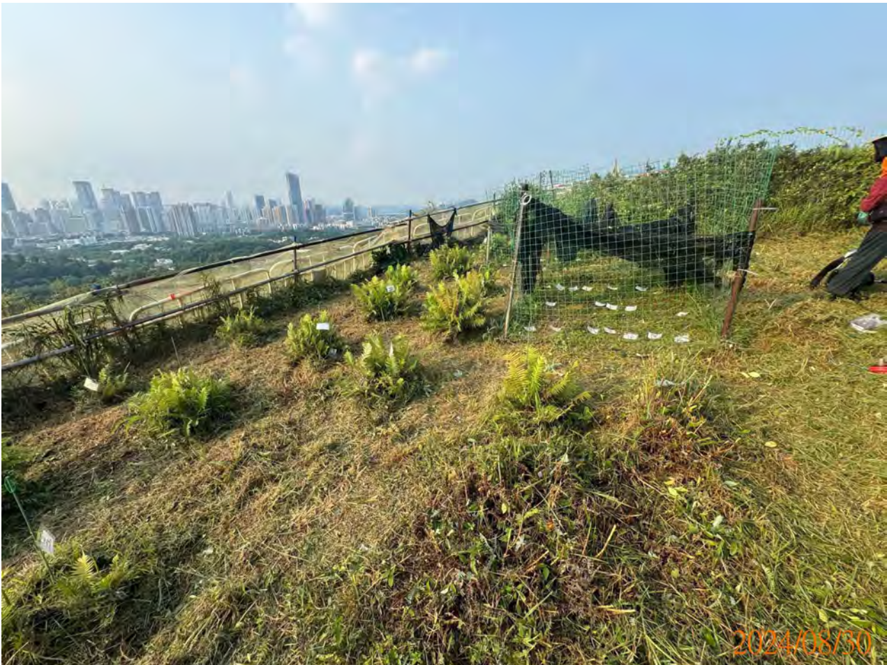
Replacement of protection fence (2)
