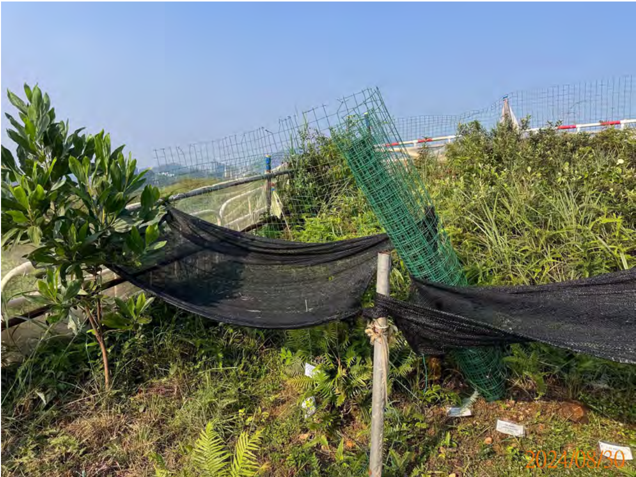
Replacement of protection fence (1)
