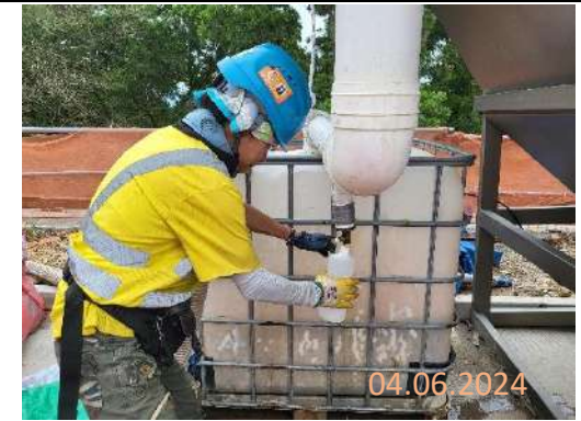
By main contractor at KNP site
