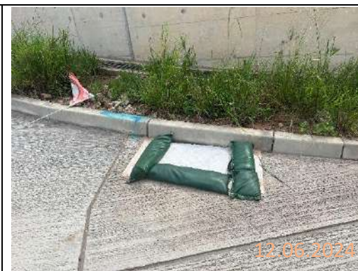
By main contractor at KNP site
