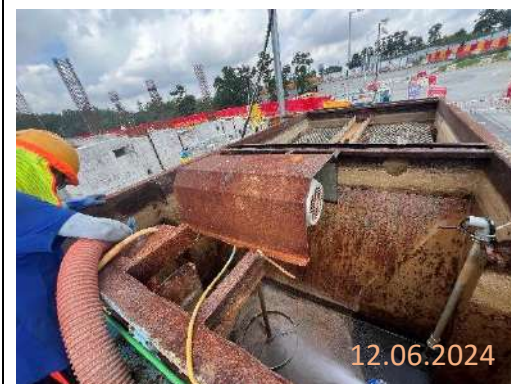
By main contractor at KNP site
