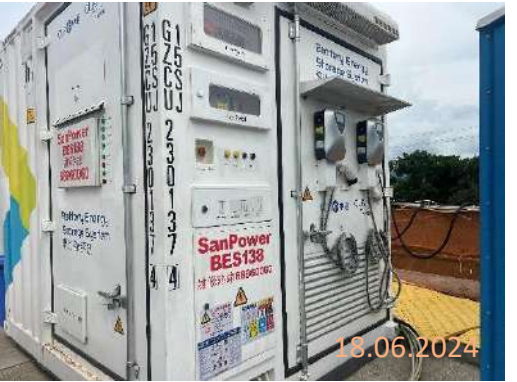
By main contractor at KNP site
