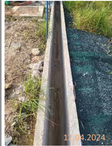
By main contractor at KNP site
