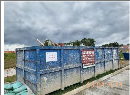
By main contractor at KNP site
