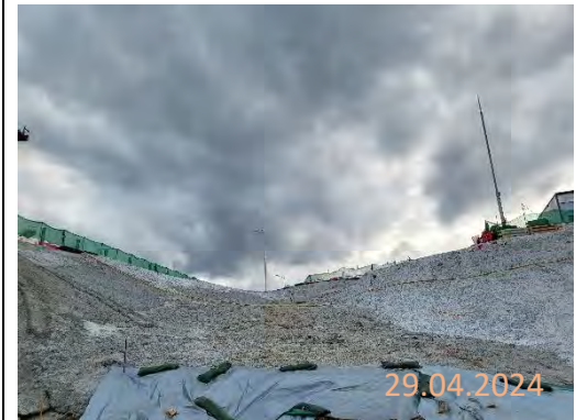
By subcontractor at KNP site
