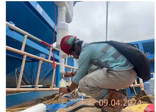
By main contractor at KNP site
