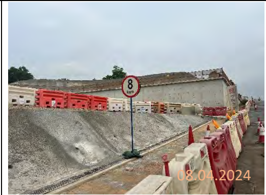
By main contractor at KNP site
