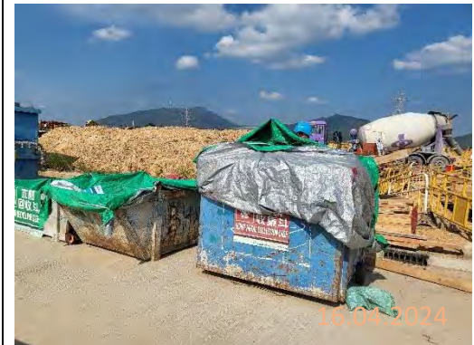
By main contractor at KNP site
