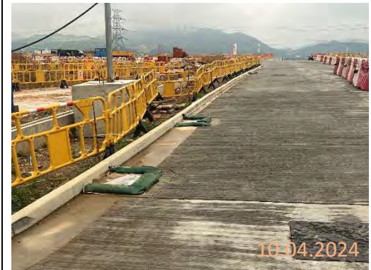
By main contractor at KNP site
