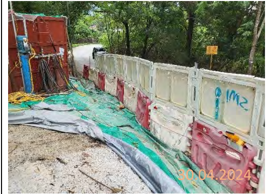
By main contractor at KNP site
