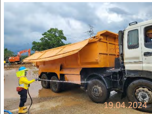
By main contractor at KNP site
