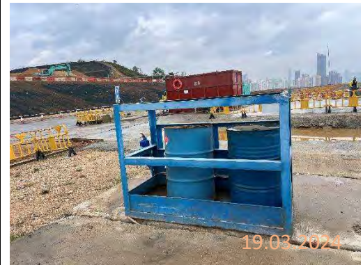
By main contractor at KNP site
