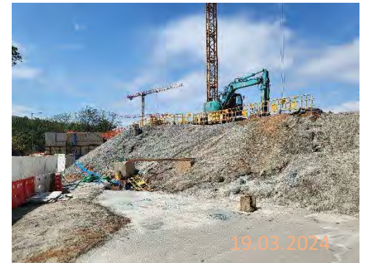
By main contractor at KNP site
