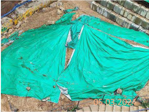
By main contractor at KNP site
