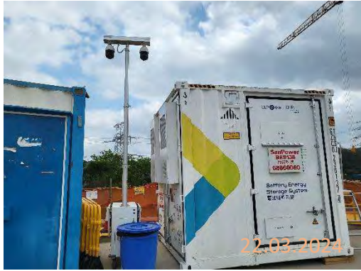
By main contractor at KNP site
