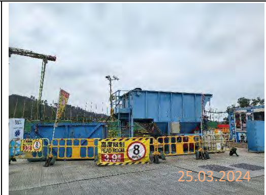
By main contractor at KNP site
