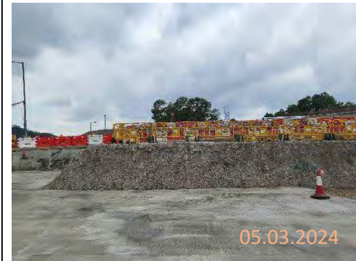
By main contractor at KNP site
