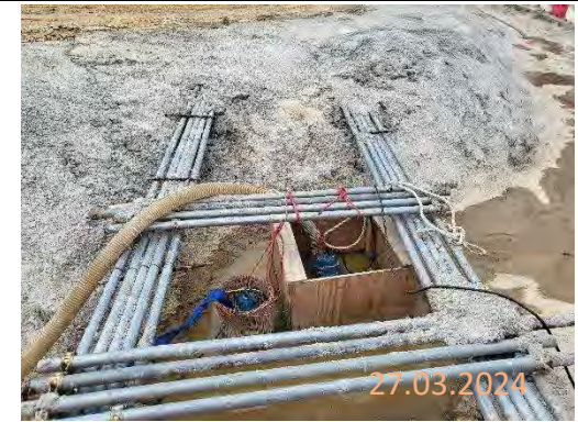
By main contractor at KNP site
