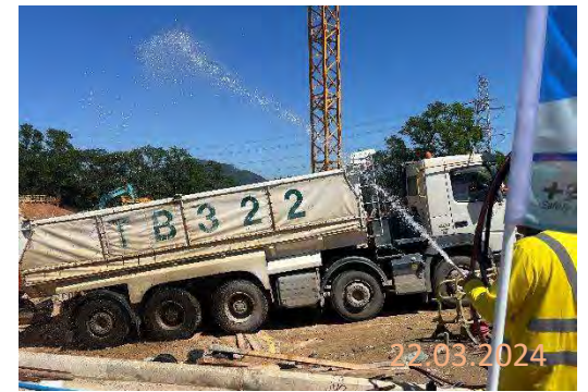
By main contractor at KNP site
