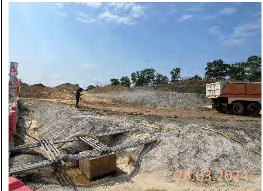
By subcontractor at KNP site
