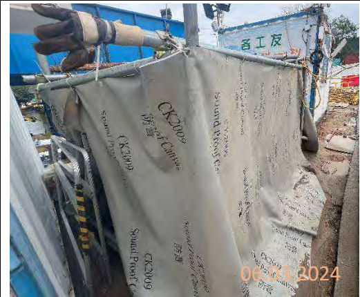
By main contractor at KNP site
