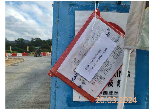
By main contractor at KNP site
