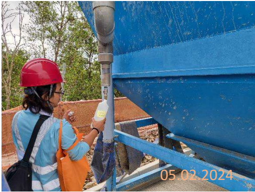
By main contractor at KNP site
