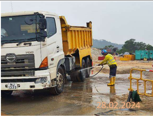
By main contractor at KNP site
