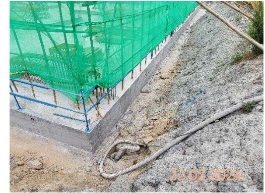
By main contractor at KNP site
