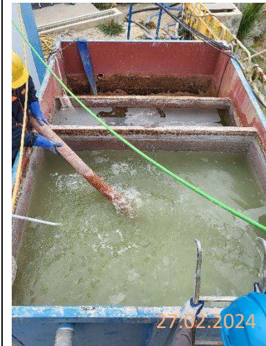
By main contractor at KNP site
