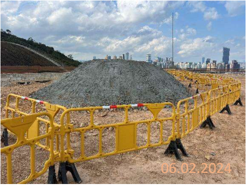
By subcontractor at KNP site
