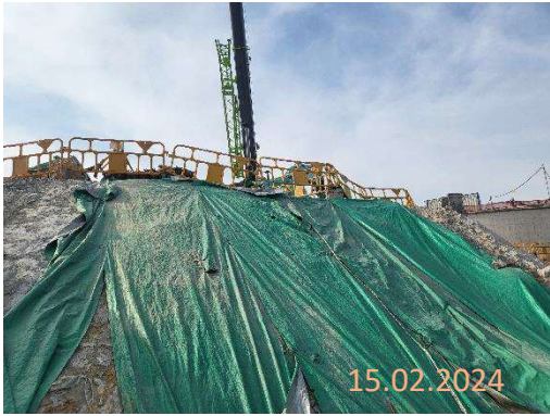
By main contractor at KNP site
