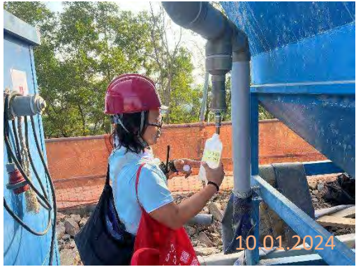
By main contractor at KNP site
