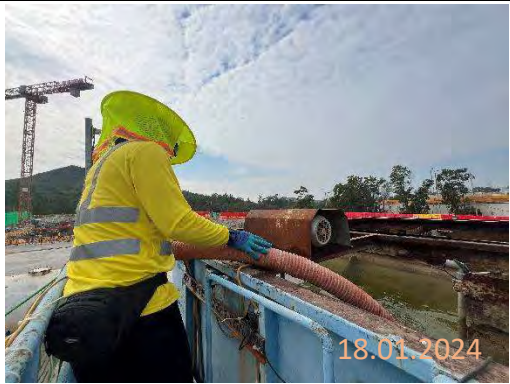
By main contractor at KNP site
