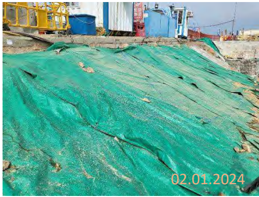
By main contractor at KNP site
