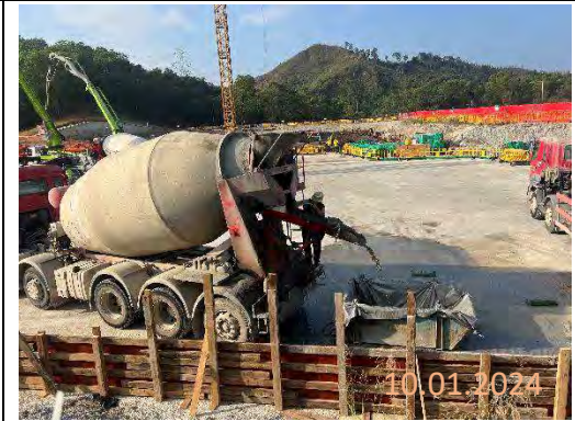
By subcontractor at KNP site
