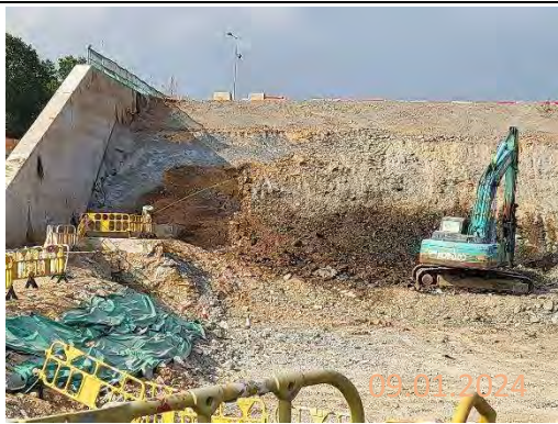
By main contractor at KNP site
