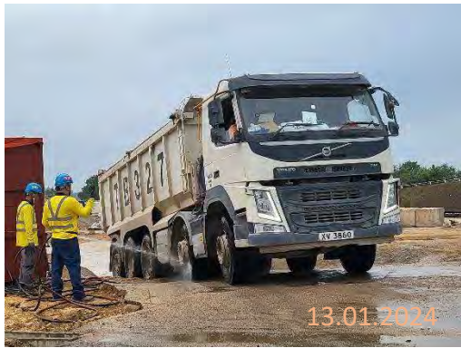
By main contractor at KNP site
