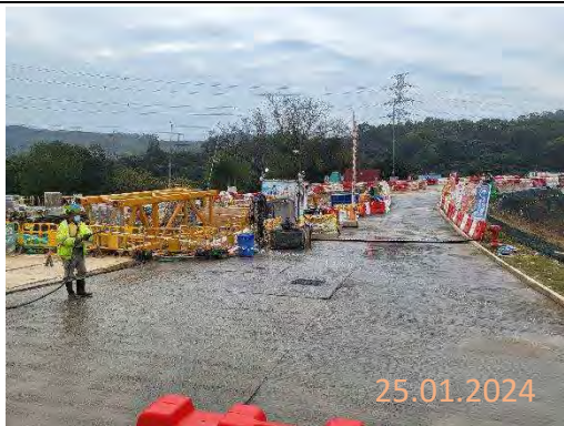
By subcontractor at KNP site
