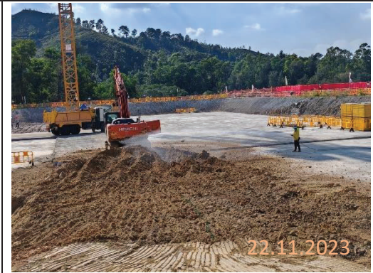
By main contractor at KNP site
