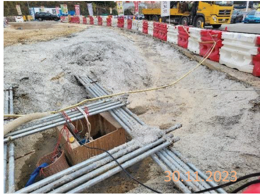
By main contractor at KNP site
