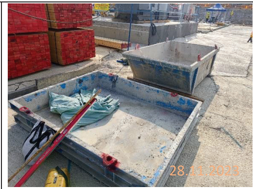
By subcontractor at KNP site
