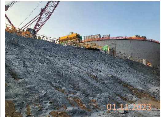
By main contractor at KNP site
