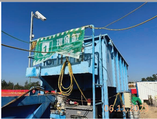
By main contractor at KNP site
