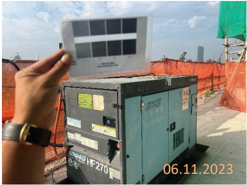
By main contractor at KNP site
