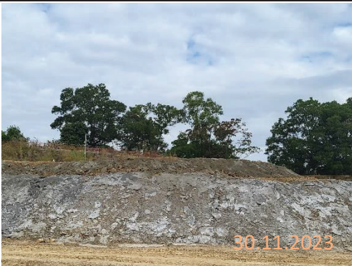
By main contractor at KNP site
