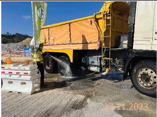
By main contractor at KNP site
