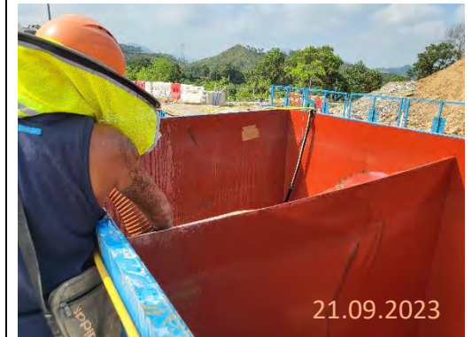
By main contractor at KNP site
