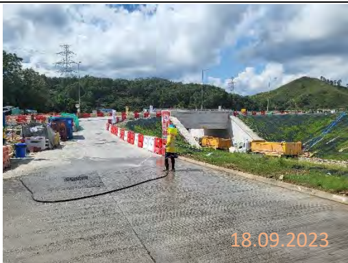
By main contractor at KNP site
