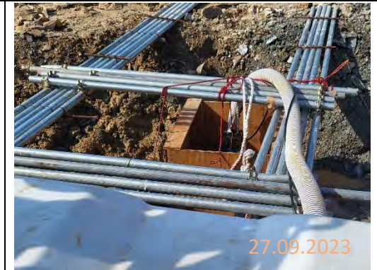
By main contractor at KNP site
