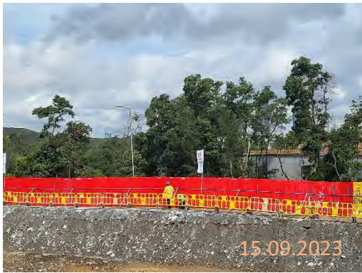
By main contractor at KNP site
