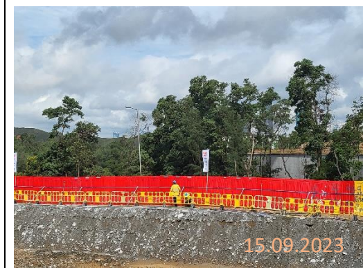
By main contractor at KNP site
