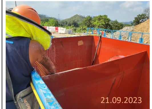
By main contractor at KNP site
