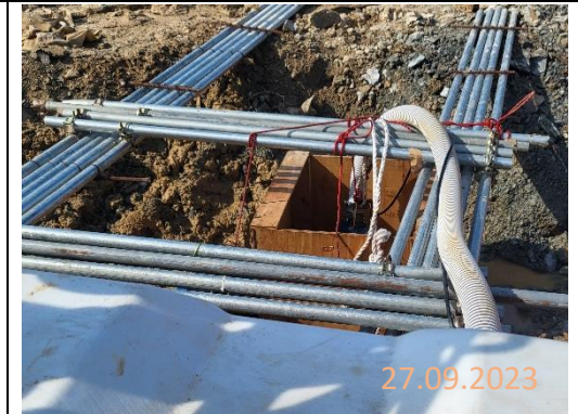
By main contractor at KNP site
