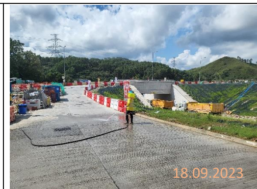
By main contractor at KNP site
