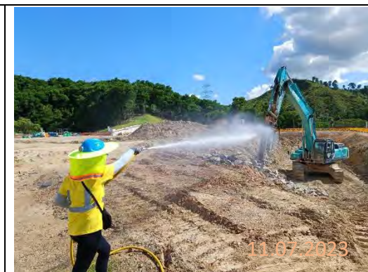
By subcontractor at KNP site
