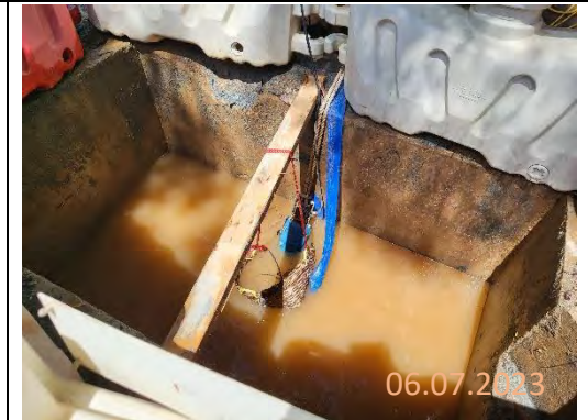
By main contractor at KNP site
