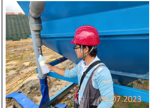
By main contractor at KNP site
