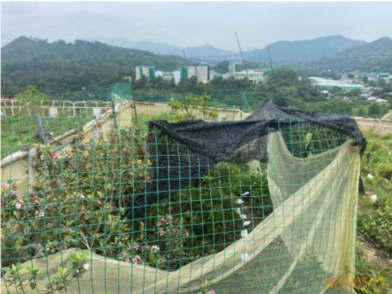
installation of shaded net (1)
