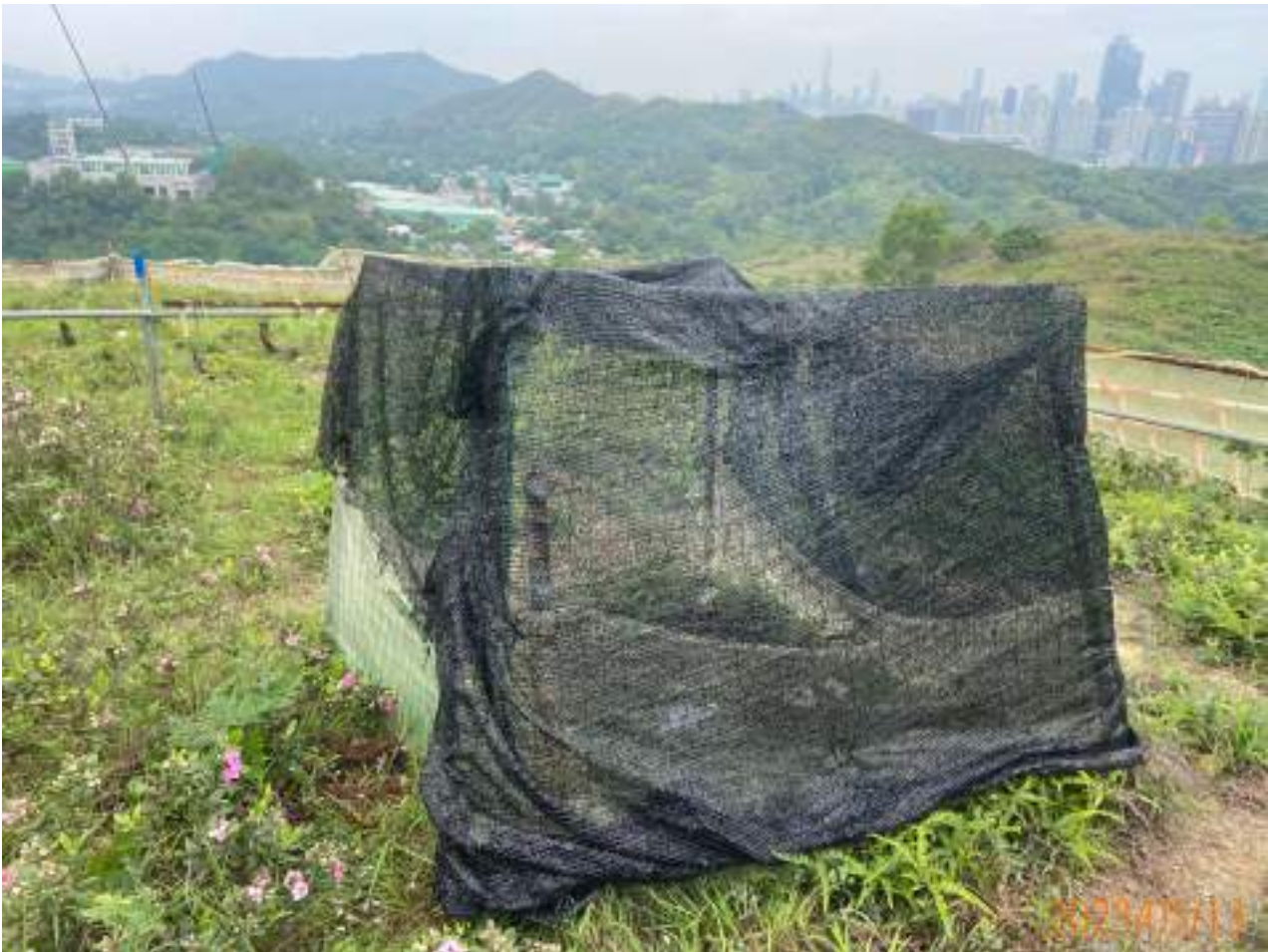
installation of shaded net (3)
