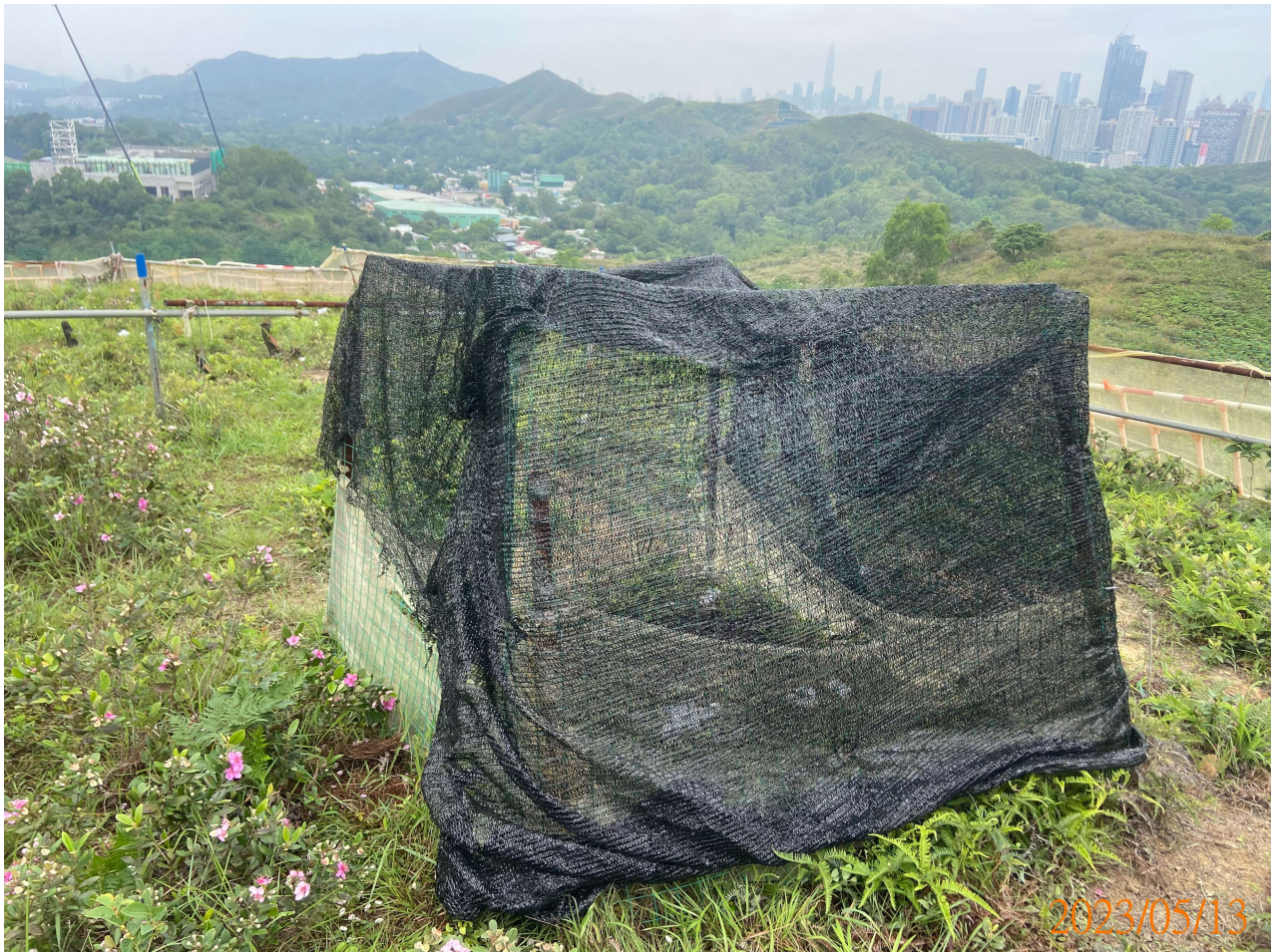
installation of shaded net (3)
