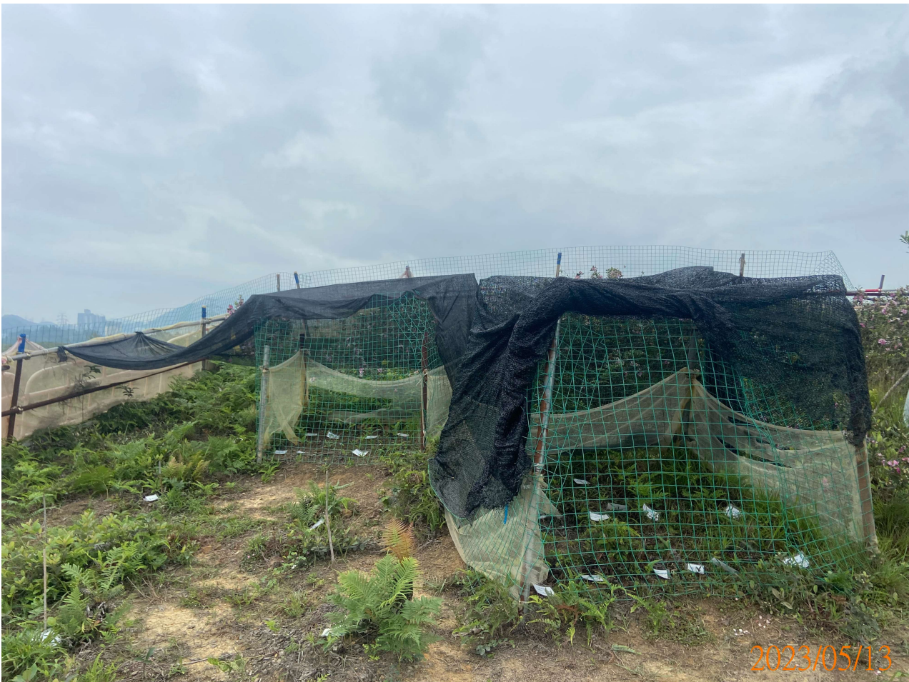
installation of shaded net (2)
