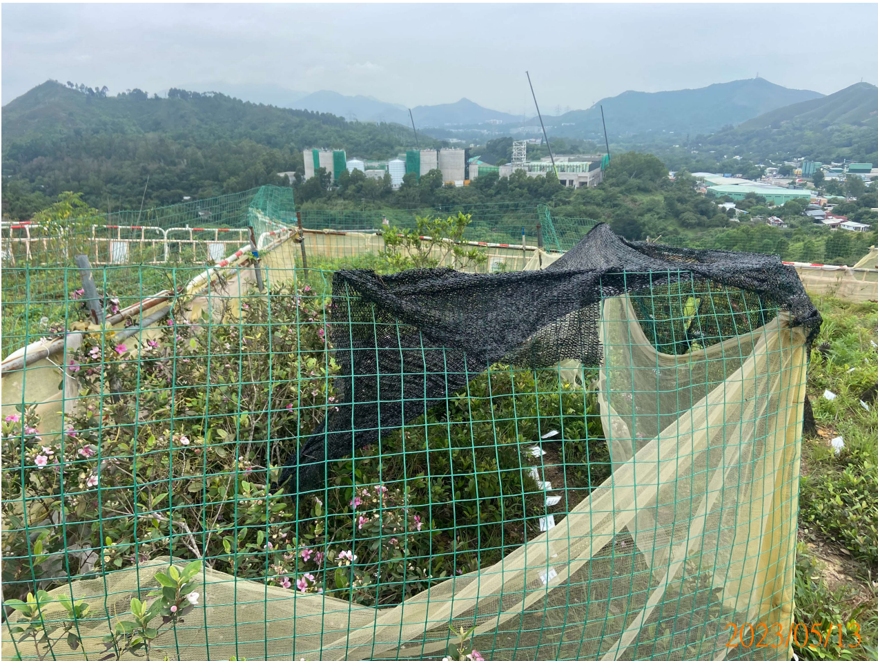
installation of shaded net (1)
