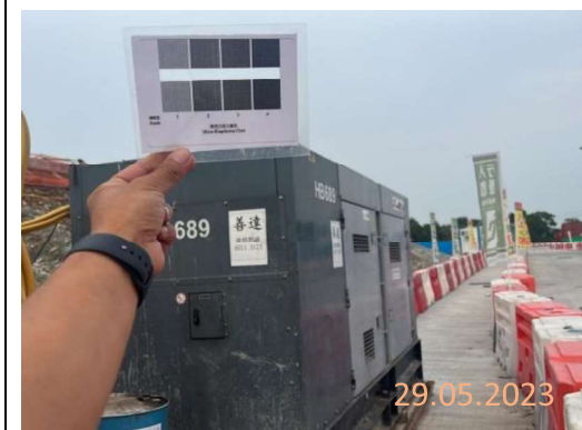
By main contractor at KNP site
