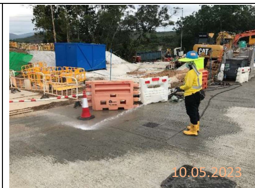
By main contractor at KNP site
